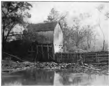
COOKSEY'S MILL, ON CLIFTY CREEK, OLDEST IN THE COUNTY
